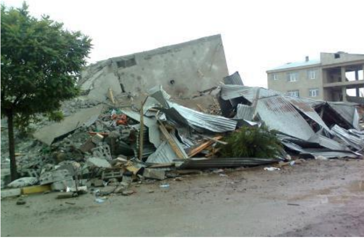
Figure3. From Van Earthquake
