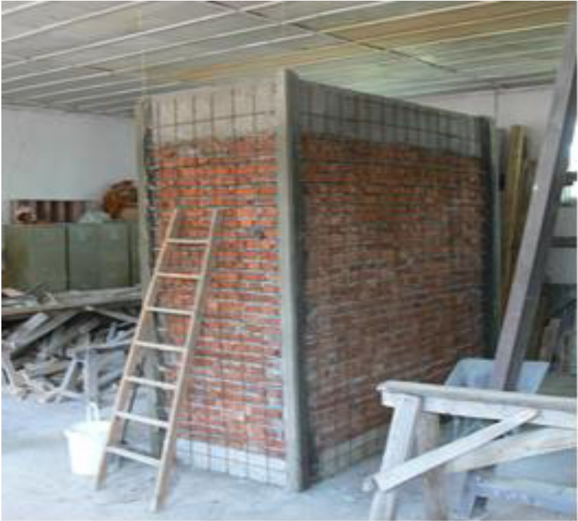
Figure 13. Covering the outer surface of the wall with steel mesh (Ateş, T.)
