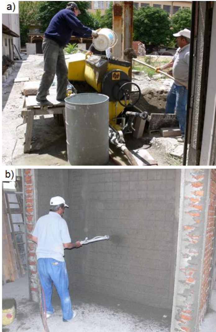
Figure 14. Spraying the inner face of the wall with shotcrete a) Preparation of concrete with ASE VP 500 TMK Shotcrete Machine b) Application of shotcrete on the inner wall of the wall (Ateş, T.)
