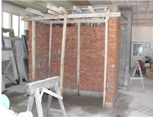
Figure 11. Wall to be covered with steel mesh (Ateş, T.)
