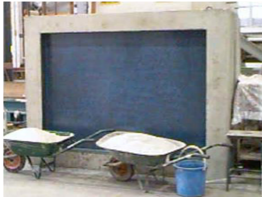
Figure 20. Strengthening the masonry wall with LTK (Coşkun, E.)
