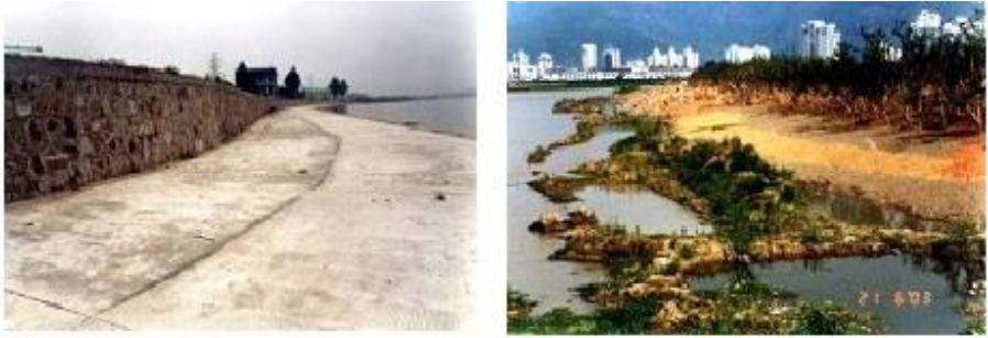
Figure 2: The Appearance of the Concrete Embankment and After Its Levelling and Transformation into A More Natural State (Kongjian & Padua, 2006)
