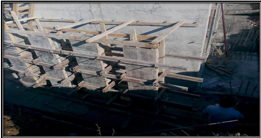
Figure 1. Concrete Forms Established For The Study
