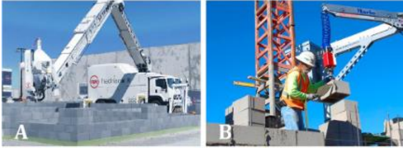
Figure 17. Robots completing a sample building (Melenbrink et al., 2020).
