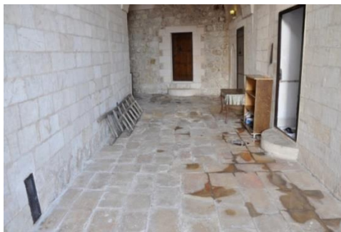
Figure 15. Efflorescence on Floor Coatings
