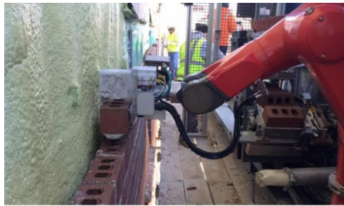
Figure 16. Brick wall robot working in site (Dakhli & Lafha, 2017)
