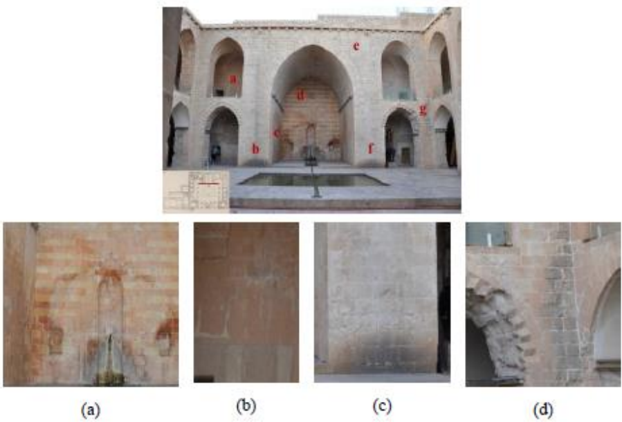
Figure 16. Deteriorations on the walls of the eastern facade of the building facing the street: change of color (a, d) defective repair (b) pitting(c)
