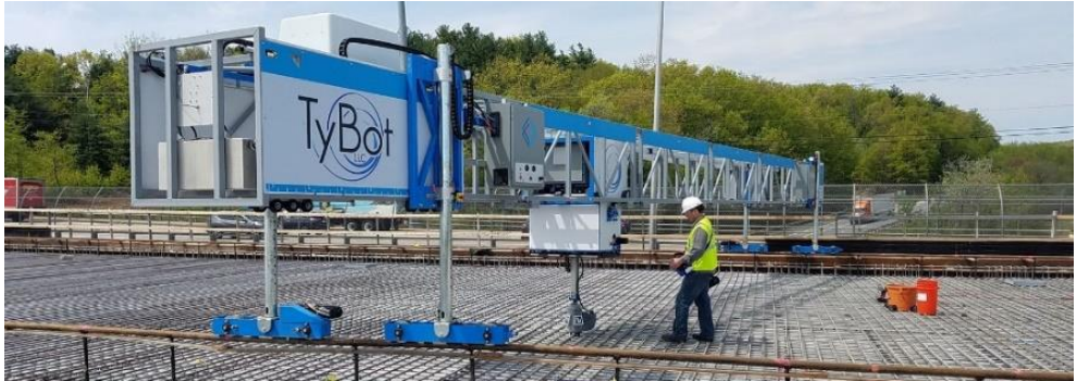
Figure 22. The robot is tying the rebars (Melenbrink et al., 2020).
