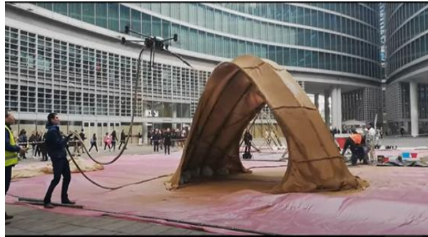
Figure 27. Bamboo structures are covered with cement with drones (Bogue, 2018).
