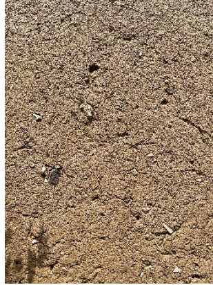
Figure 13: Detail Of Plastering With Mudbrick With High Refractory Clay Content (Baran Ergül, 2023)
