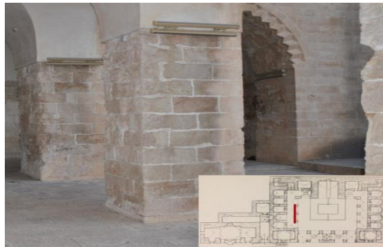
Figure 13. Defective repair on the columns
