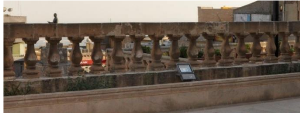
Figure 16. Surface Contamination on Railing
