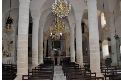
Figure 8. Efflorescence on the columns
