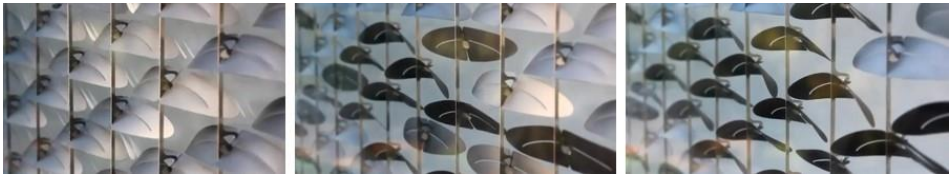
Figure 16. Motions of thermo bi-metal sheets in facade (TBM Designs, 2020)
