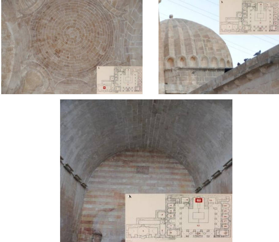
Figure 18. Change of color in the domes and vaults
