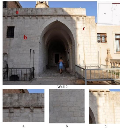
Figure 10. Material Problems on the Wall 2: a. Color Change, b. Efflorescence, c. Surface Contamination
