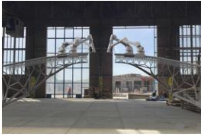
Figure 10. Robot printing the bridge (Melenbrink et al., 2020).
