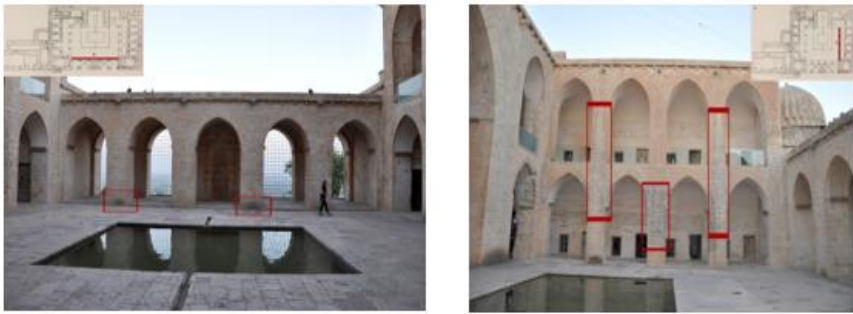
Figure 12. Change of color on the columns
