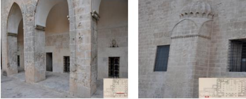
Figure 11. Loss of surface and pitting on the columns
