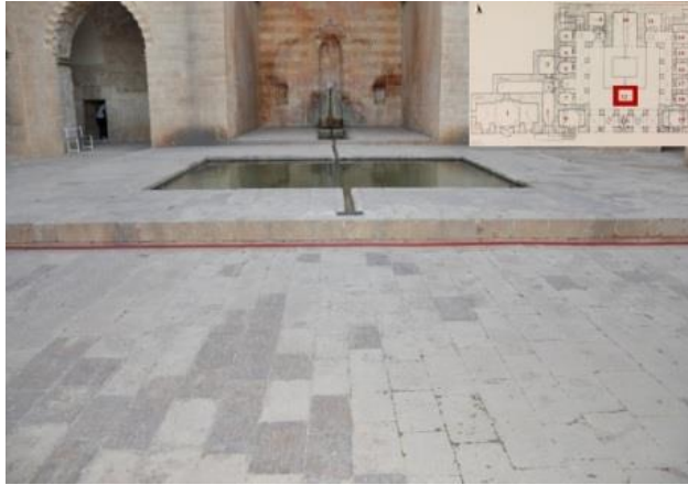
Figure 21. Change of color and tear on floor coatings
