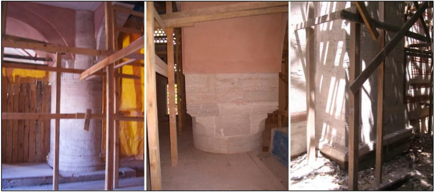
Figure 14. Circular sectioned limestone ashlar pillars with muqarnas capitals; buttress with rectangular cross-sections and limestone ashlar masonry
