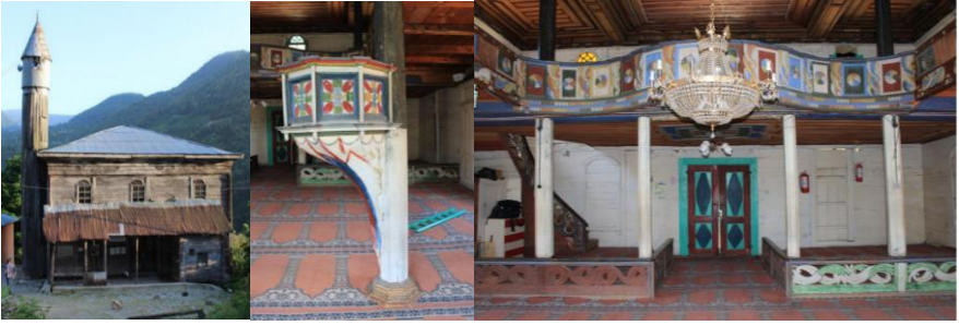
Figure 10. Macahel mosque (Zan Architecture, 2015)
