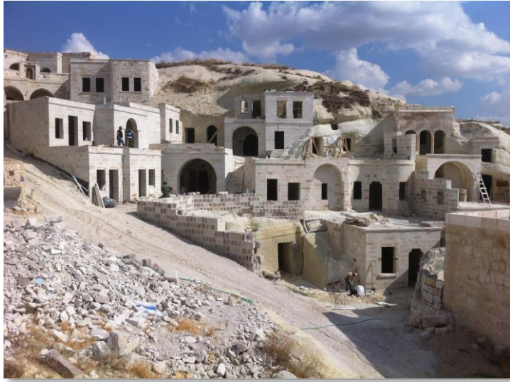
Figure 15. A dwelling converted into a hotel
