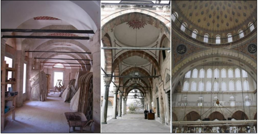
Figure 16. Arches inside the mosque and portico (of a mosque) arches The dome of the mosque; the dome with pendentives sits on a square plan (Günay, 2006). The mosque is a two-storey mosque ( fevkani ) with a rectangular plan with deep tribunes ( mahfil ) on three sides of the central space. The dome rests on the arches carried by the two piers near the front entrance door and the pillars near the mihrab (Alemdaroğlu, 1964). Dome diameter is 12.40 m and the height of the dome center is 21.80 m.
