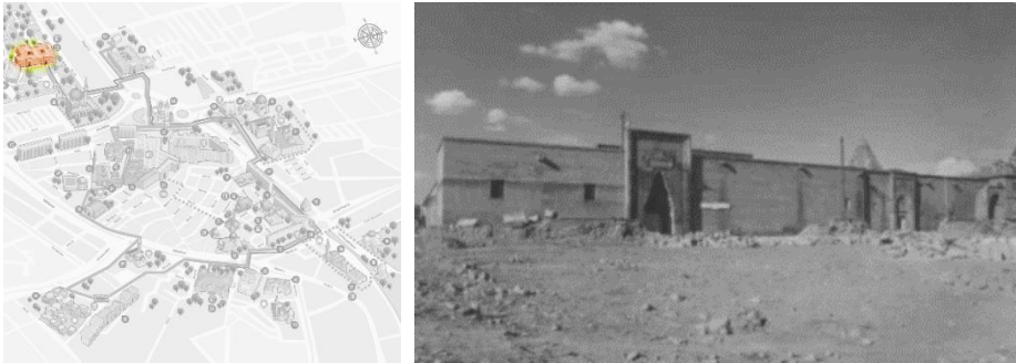
Figure 8. Gevher Nesibe Hospital and Giyasiye Madrasah on Kayseri culture route map and old photo of building (URL 8)
