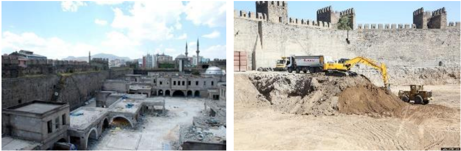
Figure 4. Construction photo of Archaeology Museum (URL 4)
