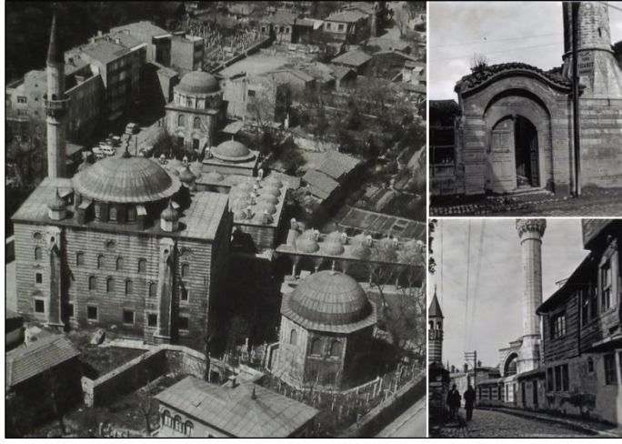
Figure 5. Photographs before the repairs
