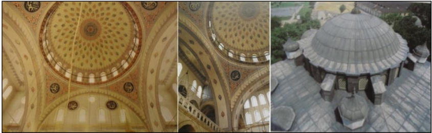
Figure 17. Dome of the mosque, dome pulley
