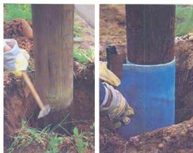
Figure 2. Application of the Bandage Method (Bozkurt, 2009)
