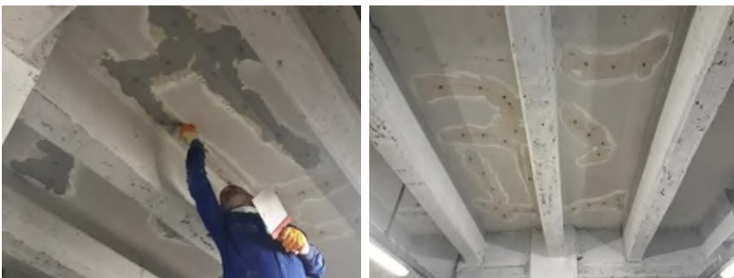
Figure 12. The Crack Repair
