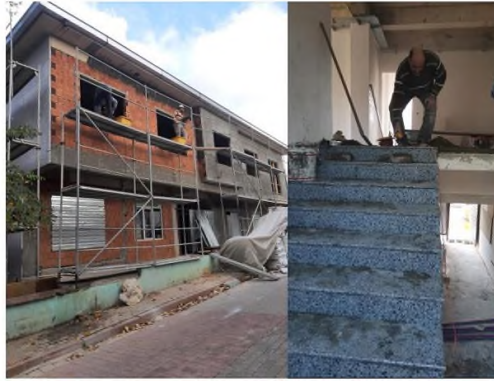
Figure 9. Various Productions During the Construction of The SHM
