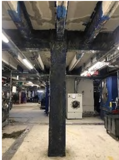
Figure 16. CFRP Application (a, b) CFRP Fabric and Laminated Reinforcement of RC Beams (c) Reinforcement of RC Columns
