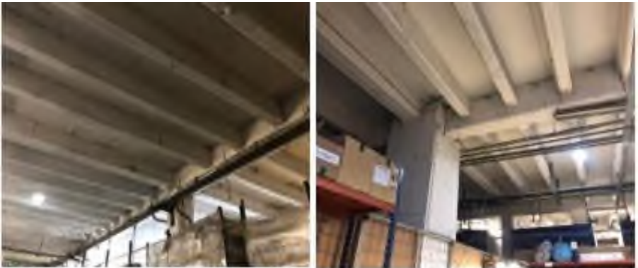
Figure 6. Existing Reinforced Concrete Industrial Structure
