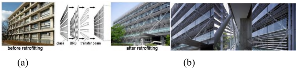
Figure 5. Tokyo Institute of Technology (TIT) Campus Retrofitting of An Existing Reinforced Concrete Building with BRBs and Façade (a) External View (b) Interior View
