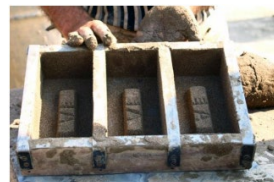
d. Kneading Mud e. Transporting the mud from the pond f. Brick mold
