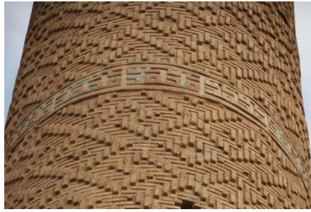
Figure 5. Hazarbaḡ Brickwork, Mudhafaria Minaret (URL, 2).
