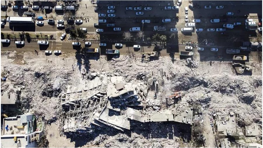
Figure 7. Urban Environment View of the February 6, 2023 Kahramanmaraş and Surroundings Earthquakes (URL-6)
