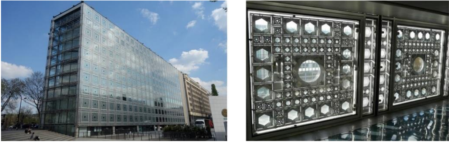
Figure 1. Facade and mechanical diaphragm detail of Institut du Monde Arabe Building (Peutz, 2023; Winstanley, 2011)
