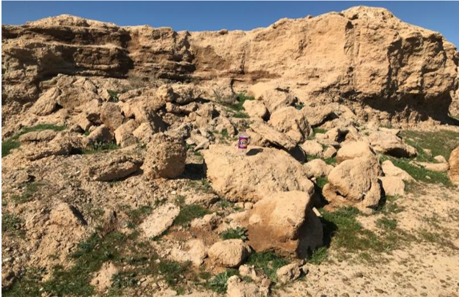
Photograph 18. Rockfall near the Al-Samtheai Village
