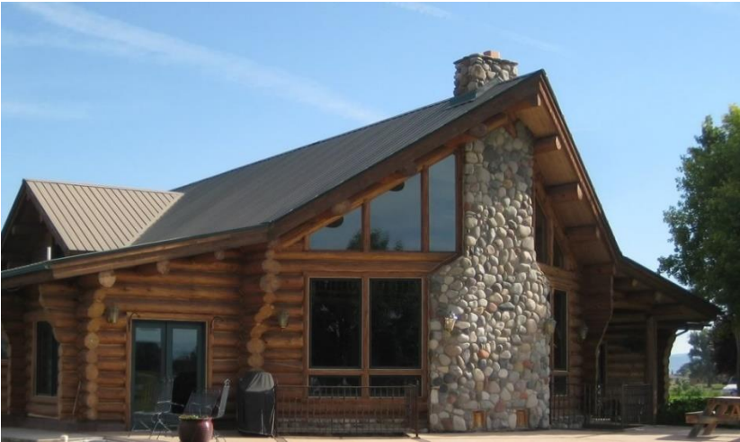
Şekil 62. Yıđma Ahşap Yapı ve Moloz Taş Duvar (Images of Completed Log Home & Cabin Construction Projects by Frontier Log Homes, 2023).
