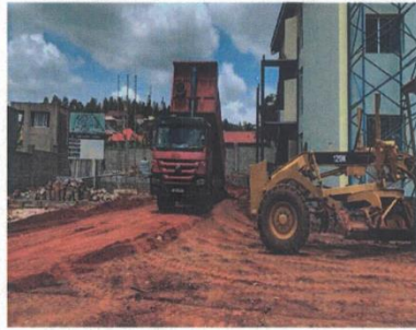
Leveling of the compound
