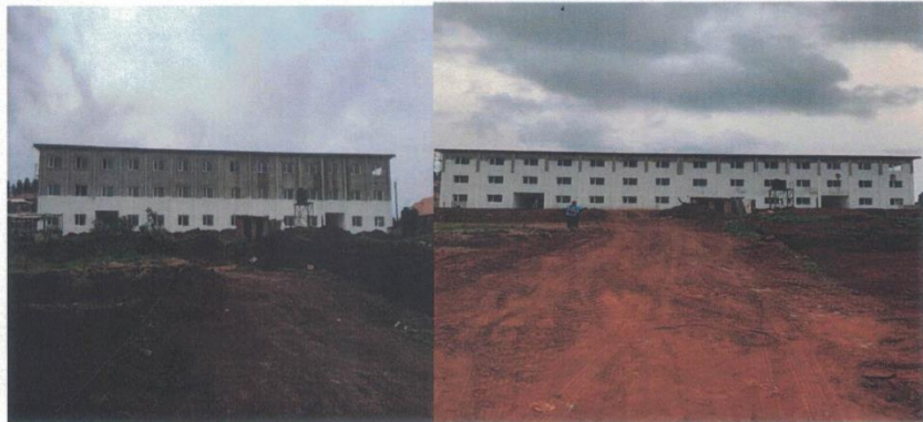
Front views of our education complex under construction by Zeta
