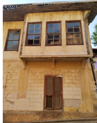
Figure 6. a., b. (top), c.,d. (middle), e., f. (bottom) Views Related to the Deteriorations Occurred in the Facade Elements of Antalya Kaleiçi Houses (Özkan Önür, 2023)
