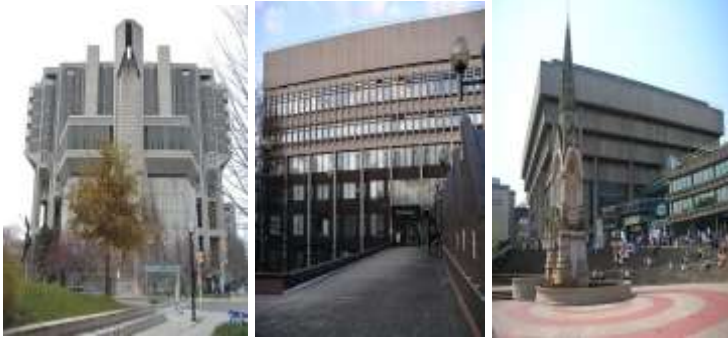
Figure 1. University of Toronto's Robarts Library, Ontario, Canada, The Coventry School of Art and Design's Graham Sutherland Building, part of Coventry University, Coventry, England, Birmingham Central Library Building, Birmingham, England, Source of image:
