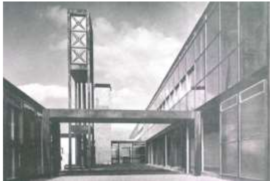
Figure 3. Hunstanton School – Norfolk, England, Peter and Alison Smithson (1949-1954) The Smithsons reduced the rationalist aesthetic of Mies van Der Rohe to an acceptable minimum, providing each element with an objective basis as a starting point for an architecture that does not the reference to nothing but itself or the function it fulfills, Source of image: https://www.architectural-review.com/buildings/school-at-hunstanton-norfolk-by-alison-and-peter-smithson
