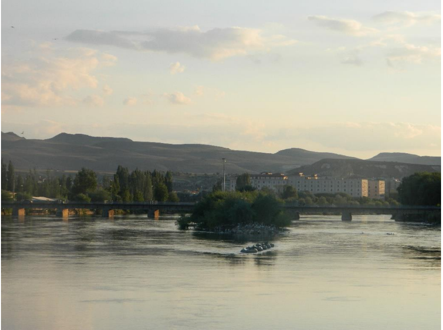
Figure 2. Avanos Historical Stone Bridge, Source: Authors
