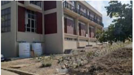
e. System in place 10.08.2022
