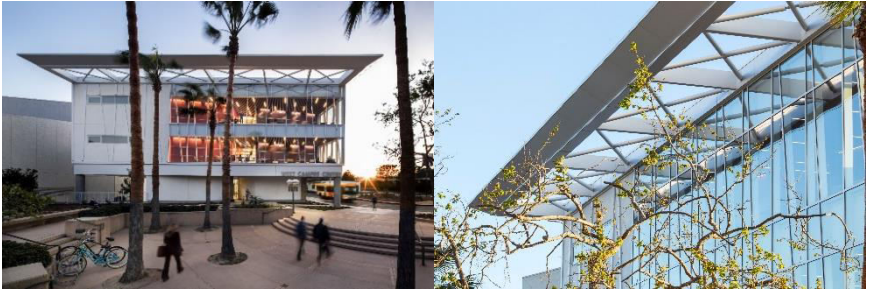
Figure 13. Wide glass facades used in the building and sunshades used as shading elements (Santa Barbara City College, n.d.)
