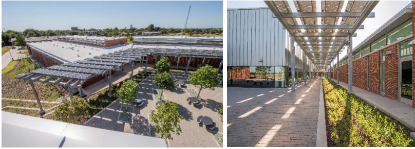
Figure 16. Solar panels providing shading effects on the building (Tarrant County College District, n.d.)
