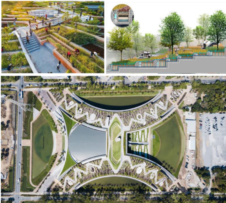
Figure 5. The largest urban rooftop farm in Asia with 22,000 m 2 green roof project located on top of Thammasat University's Rangsit Campus Building served for education and research, social responsibility, cultural landscape protection, sustainability and recreation purposes (Landprocess, 2023)
