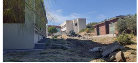
b. Removal of the concrete drainage 09.20.2022
