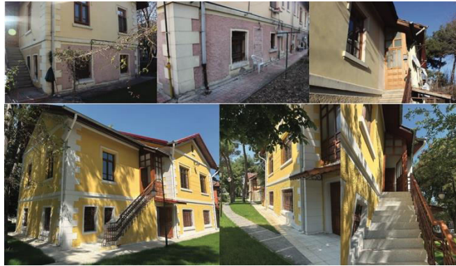
Figure 21. Exterior restorations (above: TCDD use, 2020; below: Ankara Medipol Use, 2024)
