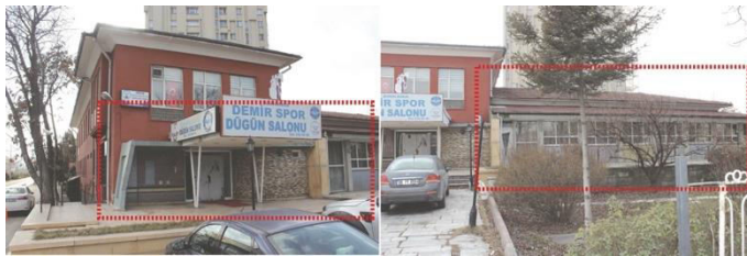
Figure 23. Additional structure, only the red structure is original
