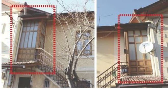
Figure 19. Entrance landings covered with glazed windows
