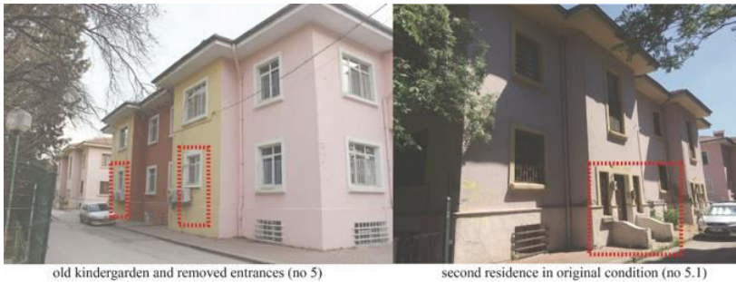
Figure 16. Original entrances of the dual officer houses
