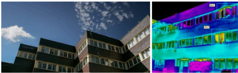
Figure 10. BMS system in Nottingham Trent University buildings (URL-6)
