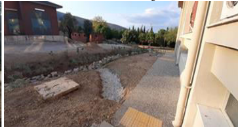
f. GI Facilities view from south 10.08.2022
