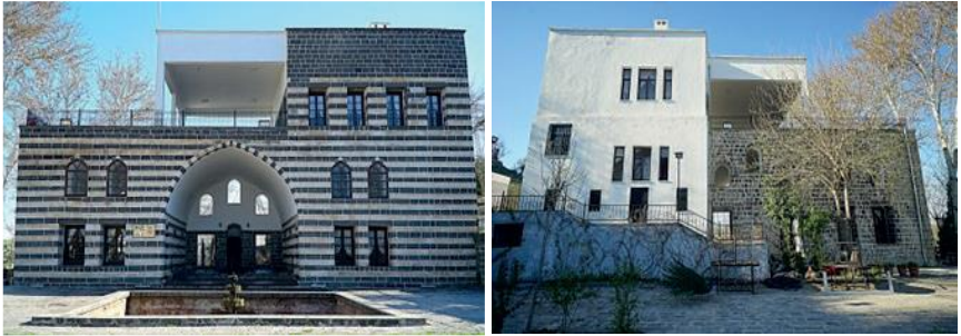
Figure 6. Gazi Mansion North and South Facade (2024)
