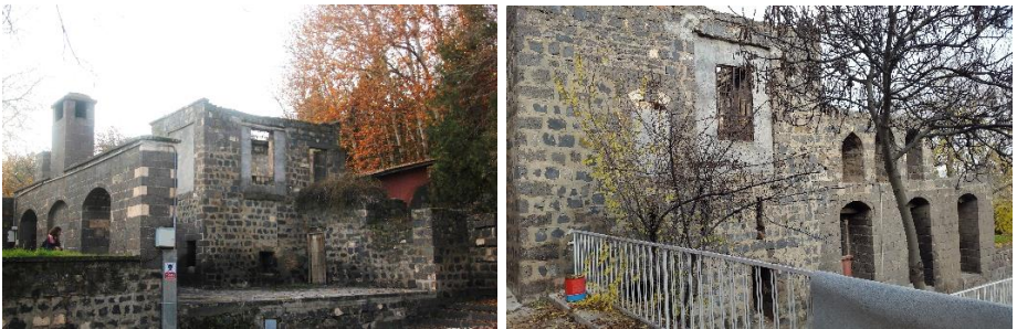
Figure 33. Demolition of the Roof and Walls in the Hami Mansion (2024)
