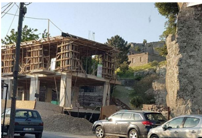
Figure 14. Assos Hotel Construction (arkeolojikhaber.com., 2024)
