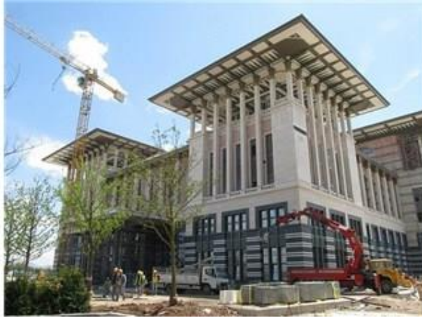
Figure 5. A public structure under construction featuring the Neo-Ottoman-Seluk Architecture
