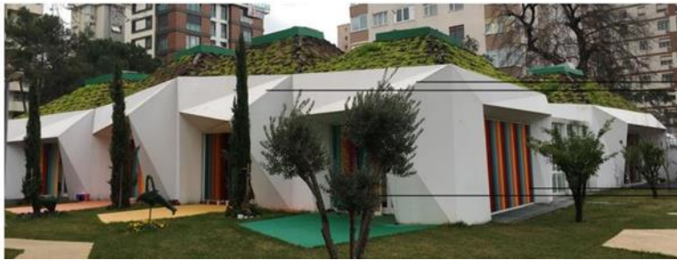
Figure 14. General view from Bahriye Üçok Kindergarten (Kızılkın & Türkyılmaz, 2021)
