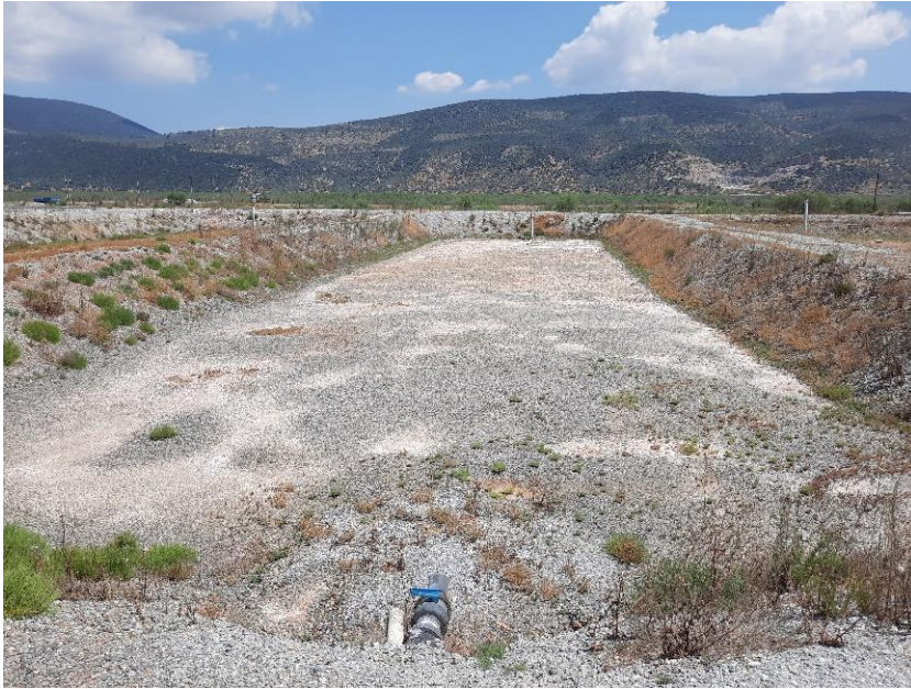
Figure 3. Earthen Pond Prepared For Use in Production
