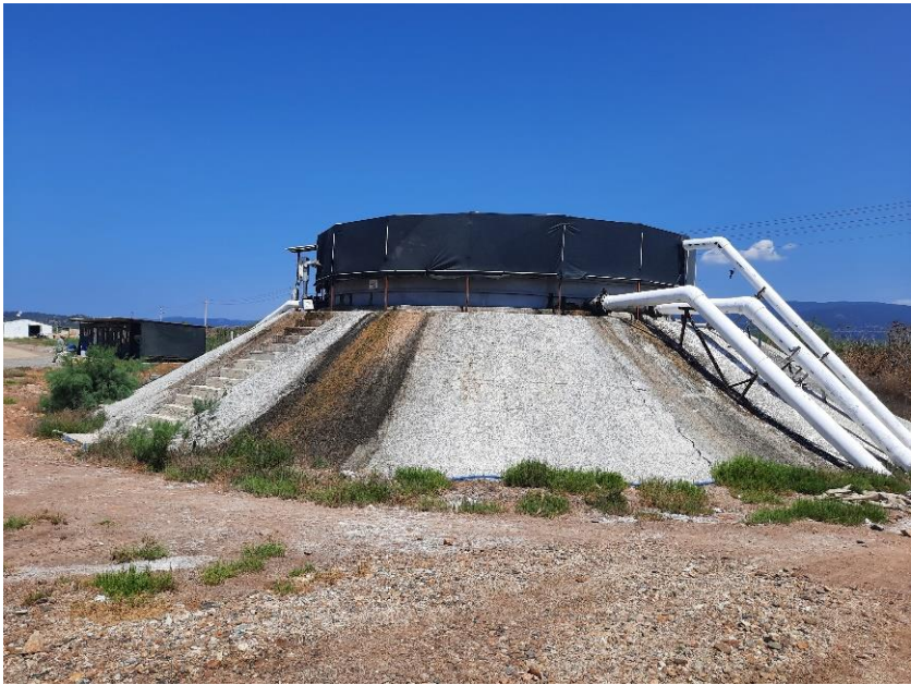
Figure 4. Water Tower Where Groundwater Is Aerated
