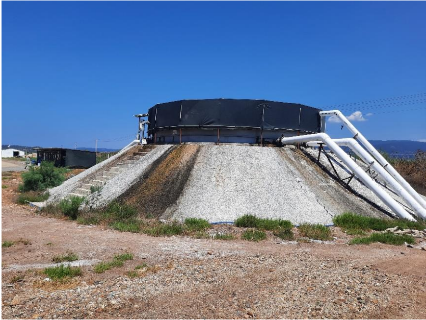
Figure 4. Water Tower Where Groundwater Is Aerated
