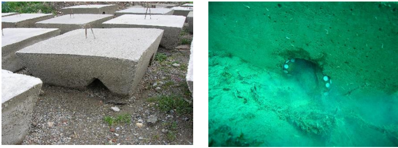
Figure 7. Construction of engineered octopus reefs (left) and their use by the octopus after deployment (right).
