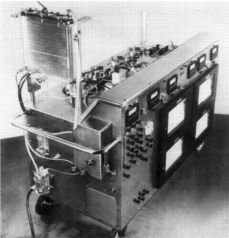
**Figure 1.** John Gibbon-IBM Co-Designed First Heart-Lung Machine
