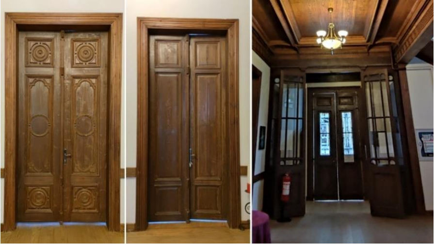
Figure 9. Doors After Cleaning and Consolidation (Osmanoğlu & Mukoviç, 2024)
