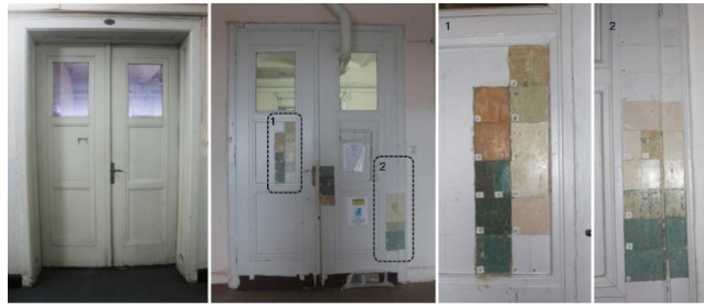
Figure 43. An example of a wooden door, showcasing its current condition and detailed stratigraphic paint layers (Osmanoğlu, 2016-2024).
