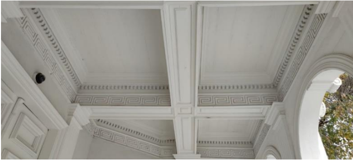
Figure 6. The condition of the balcony ceilings after restoration (Mukoviç, 2024)
