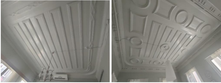
Figure 24. Ceilings of the rooms after restoration (Osmanoğlu & Mukoviç, 2024).
