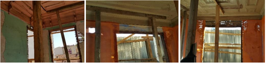
Figure 18. Suspension of the Ceilings (Osmanoğlu, 2017-2019)
