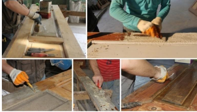
Figure 34. Mechanical and chemical cleaning applications (Osmanoğlu, 2012-2017)
