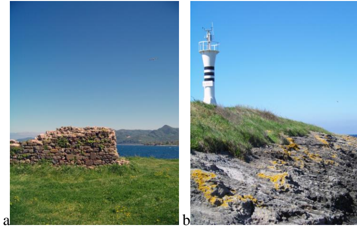
Figure 5. a) The remains of walls b) Lighthouse (Original)
