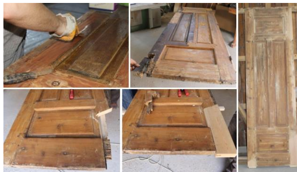
Figure 36. Details of the Consolidation Technique for Integrating Inferior Sections Following Chemical Cleaning (Osmanoğlu, 2012-2017)
