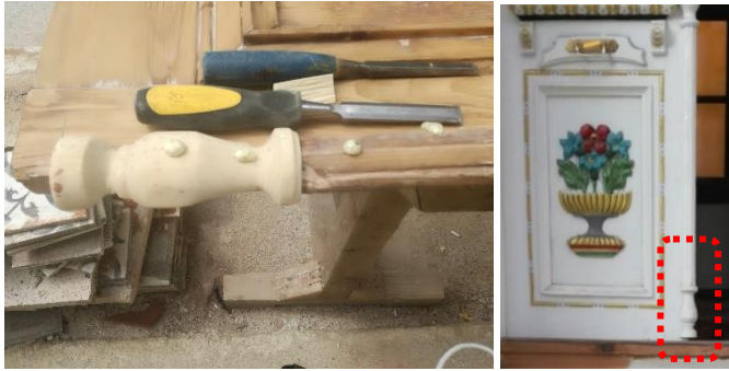
Figure 9. Application of the reintegration technique on the details of the entrance door (Osmanoğlu & Mukoviç, 2019).
