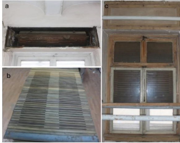
Figure 46. a) Interior of the shutter box, b) Example of the shutter during the repair process, c) Repaired shutter example installed on the window (Osmanoğlu, 2016-2024)
