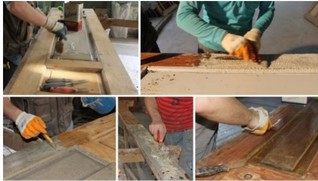
Figure 34. Mechanical and chemical cleaning applications (Osmanoğlu, 2012-2017)
