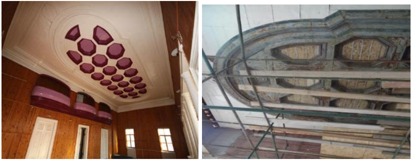
Figure 3. The conference hall's ceiling before and after restoration and stripping (Osmanoğlu, 2015).
