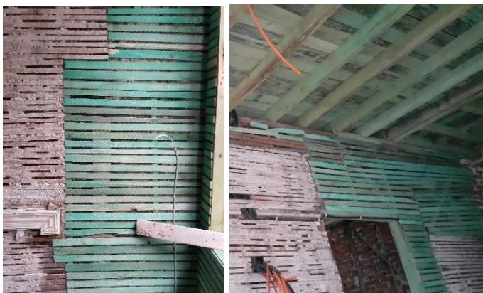
Figure 28. Application of the consolidation technique on the wattle-and-daub laths (Osmanoğlu, 2017-2019)
