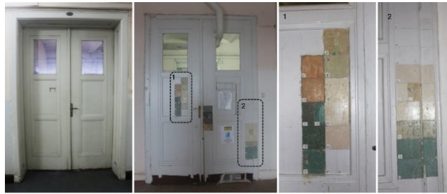
Figure 23. An example of a wooden door, showcasing its current condition and detailed stratigraphic paint layers (Osmanoğlu, 2016-2024).
