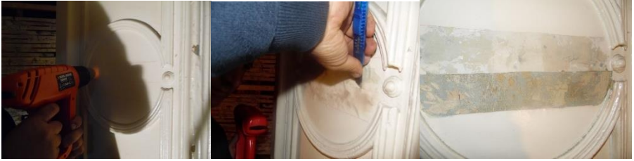
Figure 8. Cleaning Applications on the Doors (Osmanoğlu, 2015)
