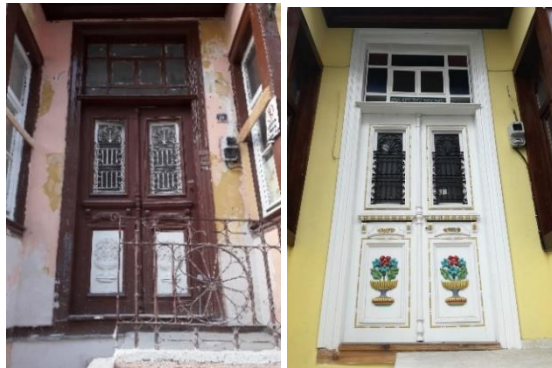
Figure 16. Entrance door before (Osmanoğlu, 2015) and after restoration (Osmanoğlu & Mukoviç, 2024)
