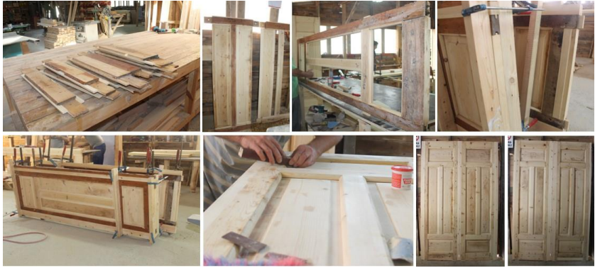
Figure 37. Disassembly of the doors and the integration of original components with newly manufactured elements using the consolidation technique (Osmanoğlu, 2012-2017)
