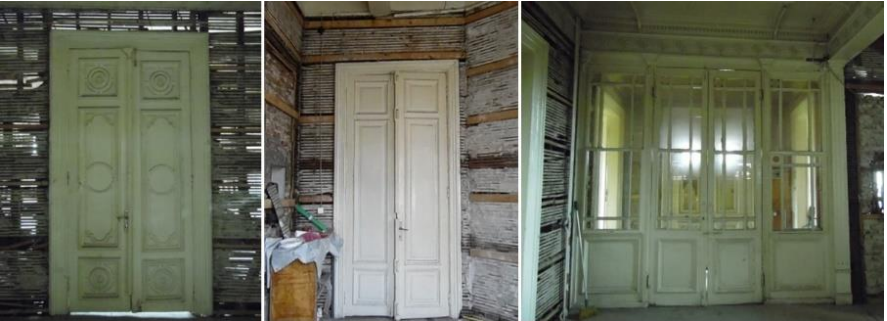
Figure 7. Doors Before Restoration (Osmanoğlu, 2015)
