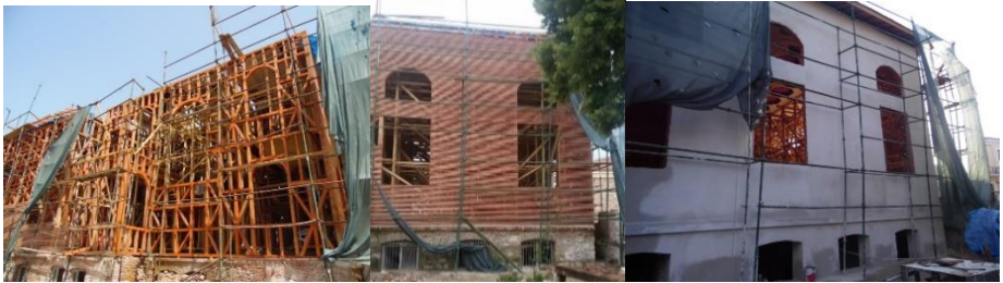
Figure 1. The restoration works included the renewal of the wooden frame system, lath strips, and plaster applications (Osmanoğlu, 2015).
