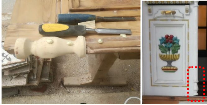
Figure 18. Application of the reintegration technique on the details of the entrance door (Osmanoğlu & Mukoviç, 2019).
