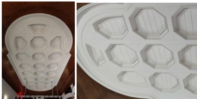
Figure 4. The conference hall ceiling after restoration (Osmanoğlu & Mukoviç, 2024)
