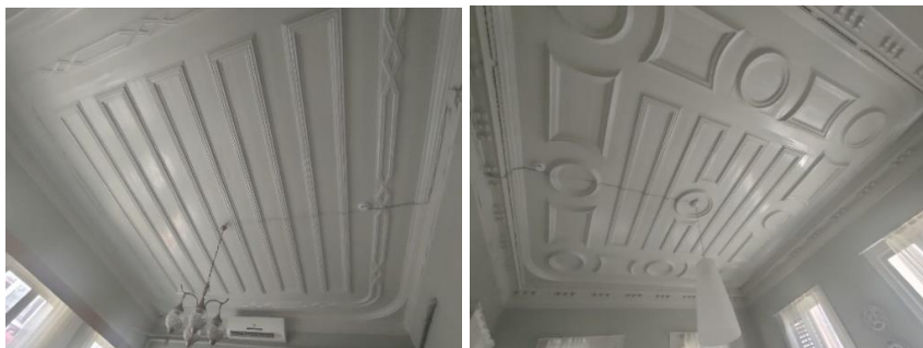
Figure 24. Ceilings of the rooms after restoration (Osmanoğlu & Mukoviç, 2024).
