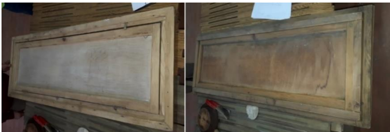
Figure 7. The front and back surfaces of the shutter box after cleaning techniques (Osmanoğlu, 2016-2024)
