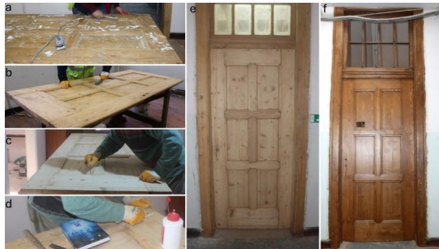
Figure 44. a) Cleaning application on the wooden door example using heat guns, b) cleaning with sandpaper, c, d) filling of gaps, e) the condition of the door after cleaning, and f) application of protective primer and varnish to the door (Osmanoğlu, 2016-2024).
