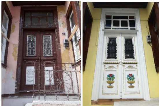
Figure 7. Entrance door before (Osmanoğlu, 2015) and after restoration (Osmanoğlu & Mukoviç, 2024)
