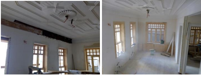
Figure 19. Interior Spaces and Ceilings Before and After Restoration (Osmanoğlu, 2017-2019)
