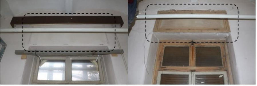
Figure 45. The condition of the shutter box lid before and after the cleaning process (Osmanoğlu, 2016-2024)
