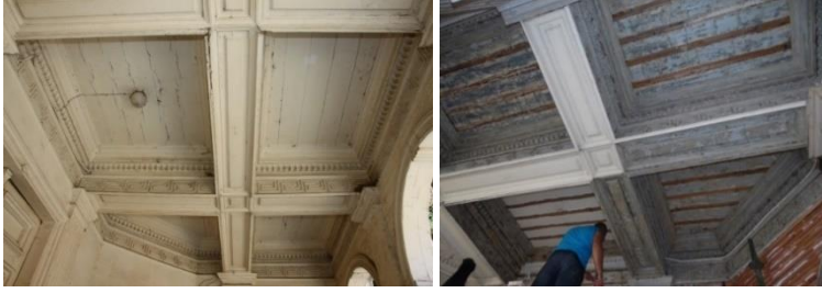
Figure 5. The condition of the building's balcony ceilings before restoration and the scraping applications (Osmanoğlu, 2015)
