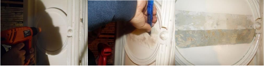
Figure 8. Cleaning Applications on the Doors (Osmanoğlu, 2015)
