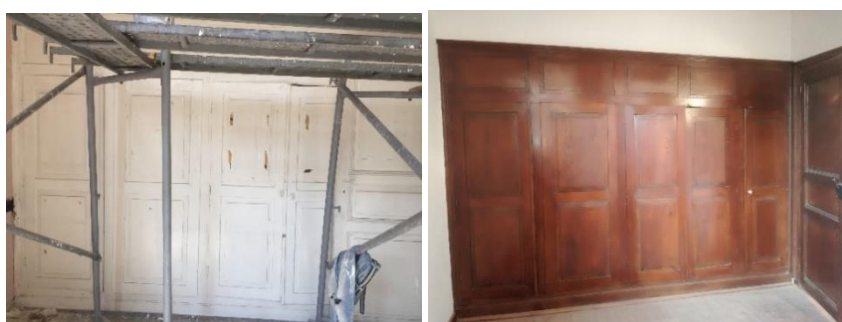
Figure 4. Ground floor original wooden cupboard before restoration (Osmanoğlu, 2015) and after restoration (Osmanoğlu & Mukoviç, 2019)
