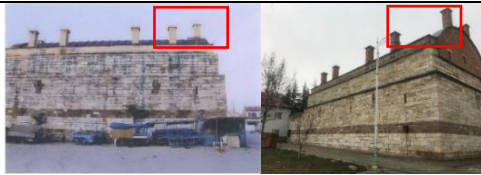
Concrete hats on the chimneys on the eastern facade of Rüstem Pasha Caravanserai before restoration (left) (restoration report, 2013) and brick hats after restoration (right)
