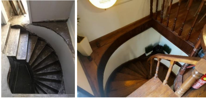
Figure 6. Staircase before restoration (Osmanoğlu, 2015) and after restoration (Osmanoğlu & Mukoviç, 2024)
