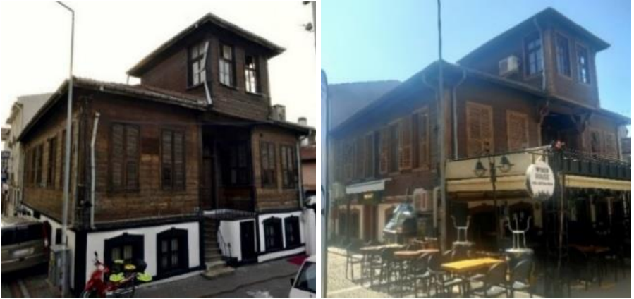
Figure 10. General appearance of the building before (Osmanoğlu, 2016) and after restoration (Osmanoğlu & Mukoviç, 2024).
