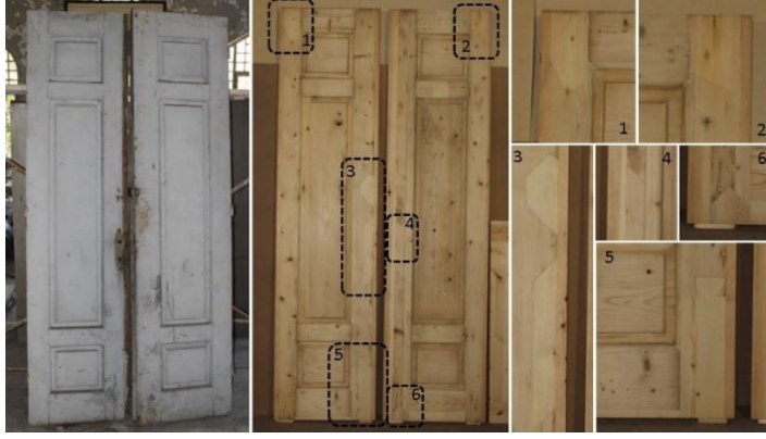
Figure 40. Ground floor door example, details of the consolidation technique 2012-2017 (Osmanoğlu)
