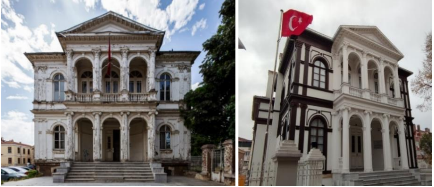
Figure 2. The appearance of the exterior before and after restoration (Osmanoğlu, 2015; Mukoviç, 2024).
