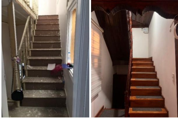
Figure 5. Staircase before restoration (Osmanoğlu, 2015) and after restoration (Osmanoğlu & Mukoviç, 2024)
