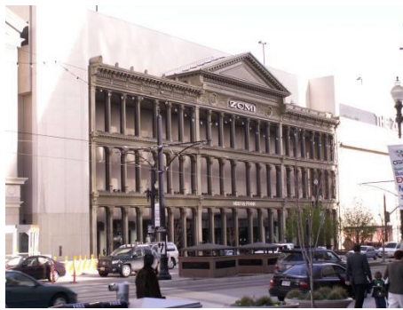
Figure 4. ZCMI Building, Salt Lake City, USA
