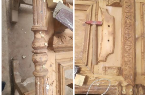
Figure 17. Cleaning processes of the entrance door (Osmanoğlu & Mukoviç, 2019).
