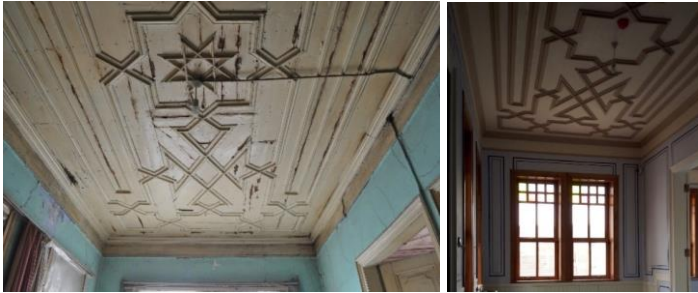
Figure 20. Interior Spaces and Ceilings Before and After Restoration (Osmanoğlu, 2017-2019)
