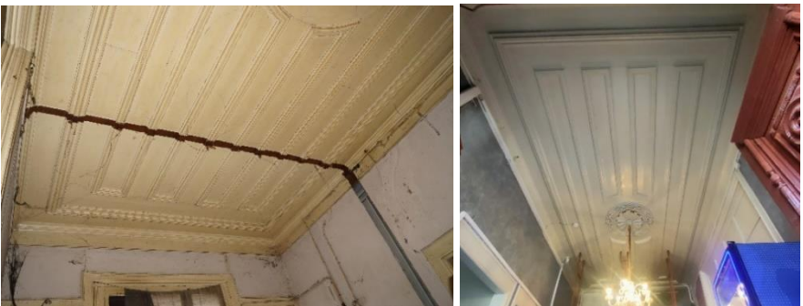
Figure 23. Restoration of the ground floor sofa ceiling before (Osmanoğlu,2016) and after restoration (Osmanoğlu & Mukoviç, 2024).
