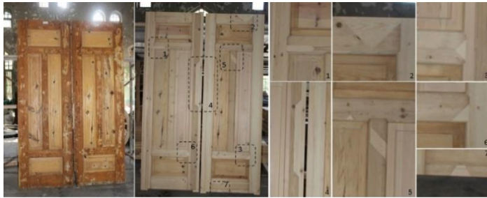
Figure 38. First floor door example, details of the consolidation technique (Osmanoğlu, 2012-2017)
