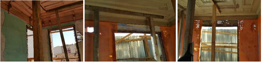
Figure 30. Suspension of the Ceilings (Osmanoğlu, 2017-2019)
