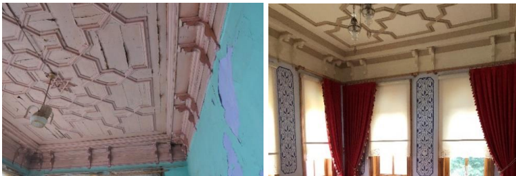
Figure 21. Interior Spaces and Ceilings Before and After Restoration (Osmanoğlu, 2017-2019)
