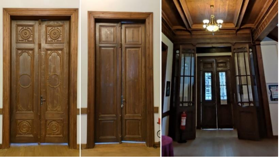
Figure 9. Doors After Cleaning and Consolidation (Osmanoğlu & Mukoviç, 2024)
