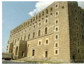
Figure 35: Aspendos Facade View (Pereira, 2007, p:50)
