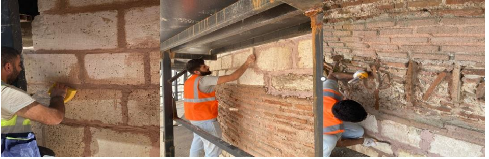
Figure 43. Consolidation applications in joint mortars, the Restoration of Macedonia Tower, Edirne, 2024, (Osmanoğlu & Köse, 2024)
