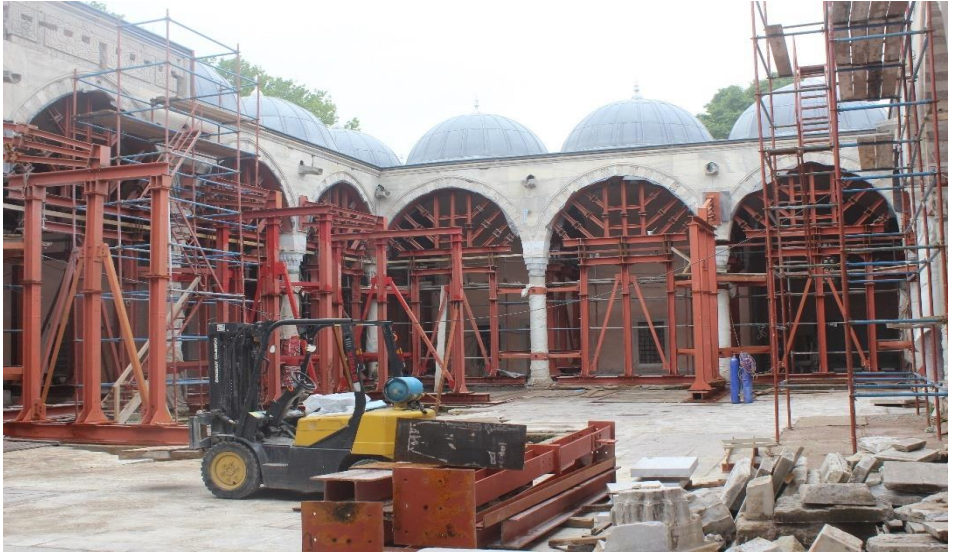
Figure 14. Application of suspension for the repair of the columns in the porticoes of the courtyard, Restoration of Tabhane Building of Süleymaniye Complex, Istanbul, 2012-2018, (Osmanoğlu, 2014)
