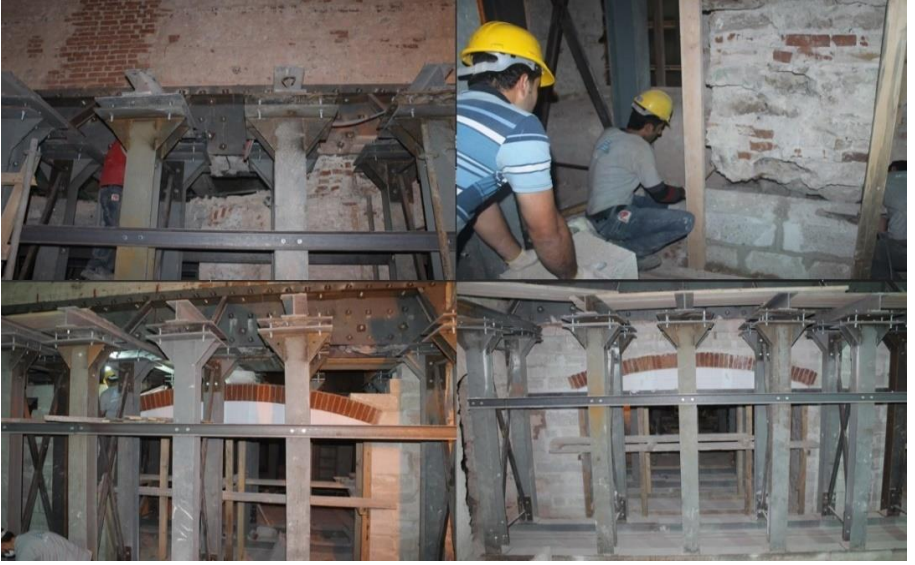
Figure 26. Suspension works of the basement supporting columns for repair procedures, Restoration of Fatih Sultan Mehmet High School, Istanbul, 2010-2017, (Osmanoğlu, 2010)
