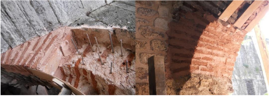
Figure 19. Removal of bricks that have lost their strength in the arches and application of anchorage with epoxy resin and steel rods for the installation of newly produced original bricks, Restoration of Tabhane Building of Süleymaniye Complex, Istanbul, 2012-2018, (Osmanoğlu, 2013)
