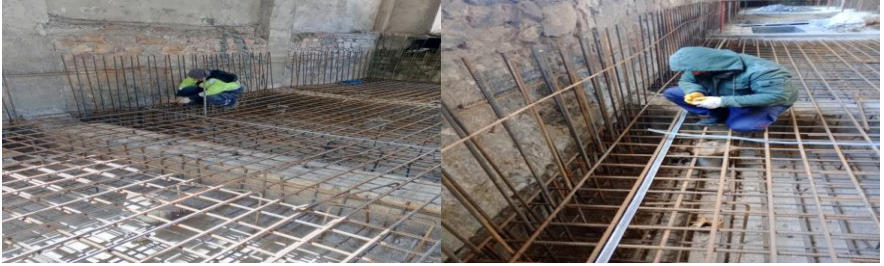
Figure 35. Anchoring of the piles and raft foundation reinforcements created to remain above the existing foundation, Restoration of the Building No. 5, Haydarpaşa Train Station, Istanbul, 2017-2024, (Osmanoğlu, 2017)
