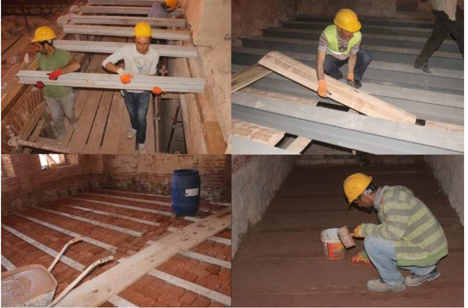
Figure 33. Reinforcement and consolidation applications on arch ceilings with reduced load-bearing capacity due to section loss in iron profiles and damage to the bricks forming the arch, Restoration of Fatih Sultan Mehmet High School, Istanbul, 2010-2017, (Osmanoğlu, 2016)
