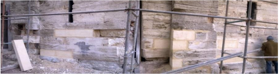
Figure 11. Stitching operation on stone walls, Restoration of Darüşşifa Building of Süleymaniye Complex, Istanbul, 2009-2016, (Osmanoğlu, 2010)
