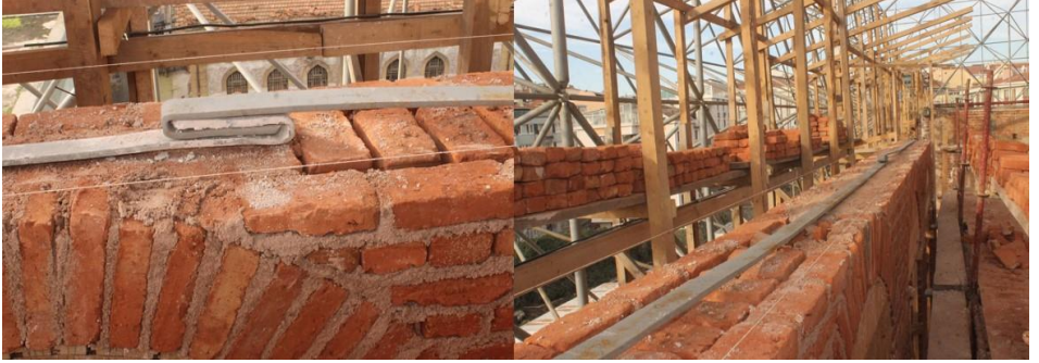
Figure 32. Reinforcement along the length of the wall beneath the supporting steel beams of the arch ceiling, Restoration of Fatih Sultan Mehmet High School, Istanbul, 2010-2017, (Osmanoğlu, 2015)
