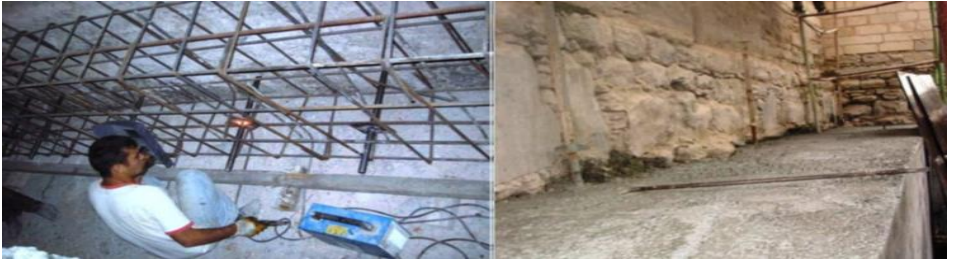
Figure 3. Reinforcement application using reinforced concrete for the foundations, Restoration of the Bayezid II Bath, Istanbul, 2005-2014, (Osmanoğlu, 2006)
