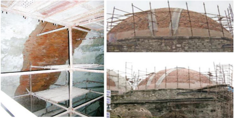
Figure 1. Repair of cracks in the right main dome of the Bayezid II Bath through stitching method, reinforcement application with carbon fiber tape in the left main dome, Restoration of the Bayezid II Bath, Istanbul, 2005-2014, (Osmanoğlu, 2008)
