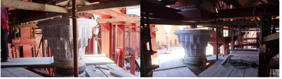
Figure 15. Installation of the repaired column capital, Restoration of Tabhane Building of Süleymaniye Complex, Istanbul, 2012-2018, (Osmanoğlu, 2014)
