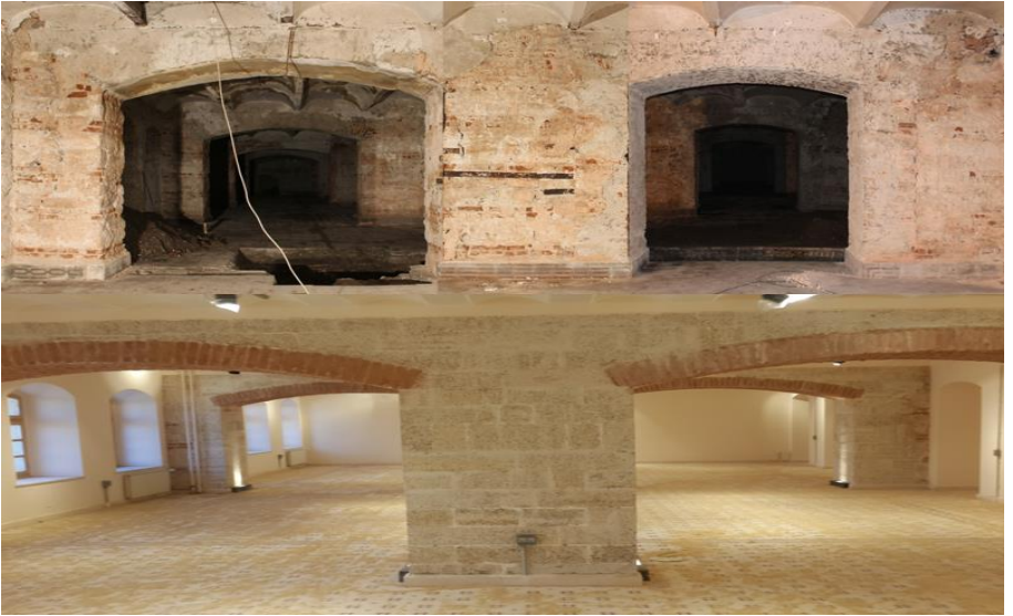
Figure 27. Before and after conditions of consolidation and reinforcement works on the basement columns, Restoration of Fatih Sultan Mehmet High School, Istanbul, 2010-2017, (Osmanoğlu, 2010-2017)
