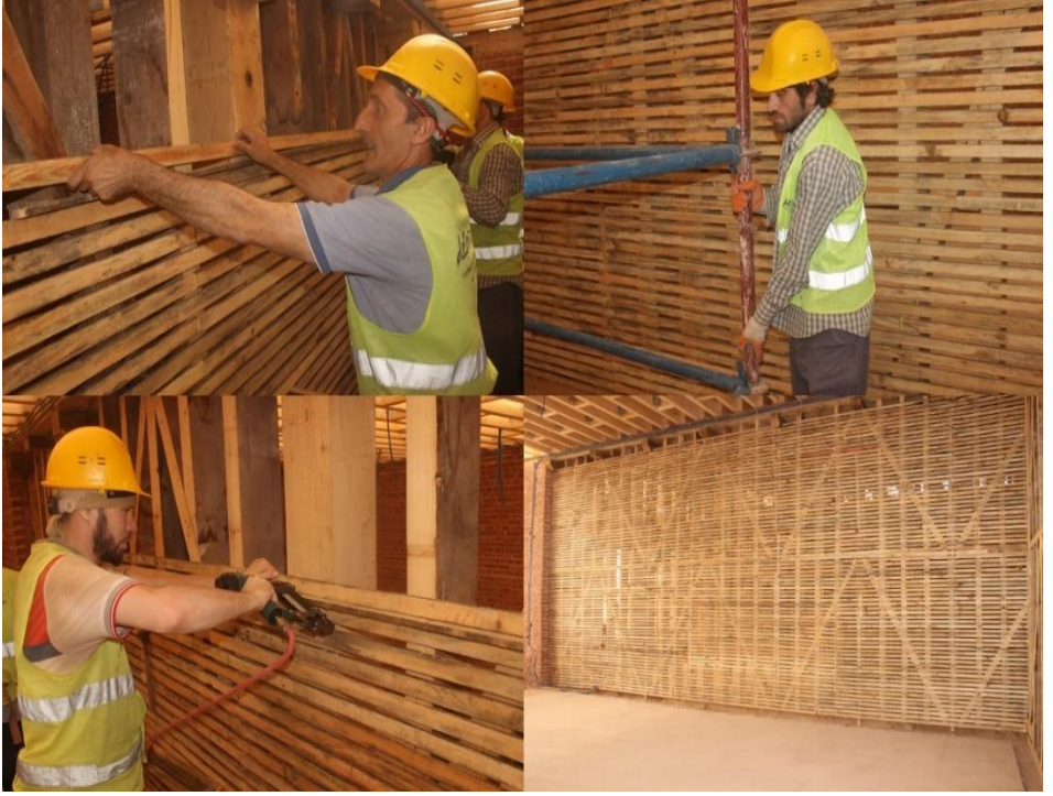
Figure 28. Repair of damaged and weakened wooden structural elements and lath, Restoration of Fatih Sultan Mehmet High School, Istanbul, 2010-2017, (Osmanoğlu, 2012)
