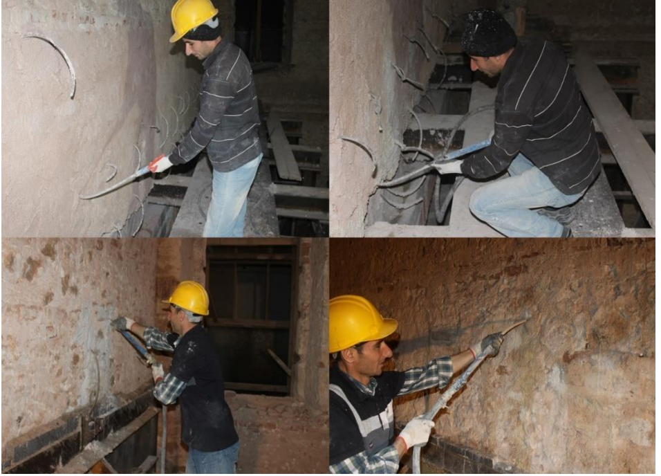
Figure 30. Hydraulic lime injection applications to cracks and voids in the walls, Restoration of Fatih Sultan Mehmet High School, Istanbul, 2010-2017, (Osmanoğlu, 2012)
