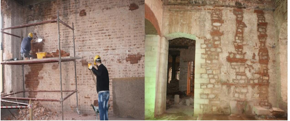
Figure 31. Removal of damaged and unusable bricks due to structural damage and stitching applications made with original forms, materials, and techniques, Restoration of Fatih Sultan Mehmet High School, Istanbul, 2010-2017, (Osmanoğlu, 2012)
