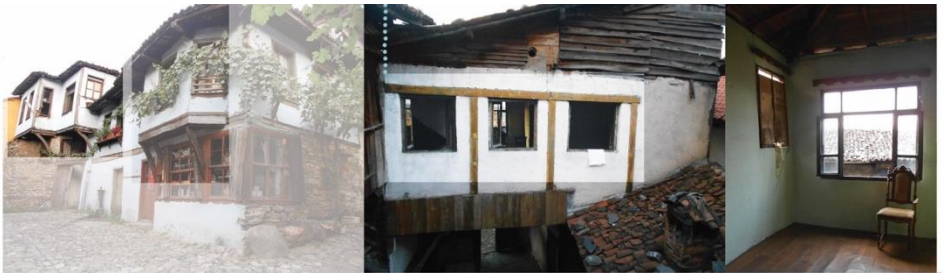
Figure 11. Projections Extending from Room to Courtyard and from Courtyard to Street (Adigüzel Özbek, 2015).
