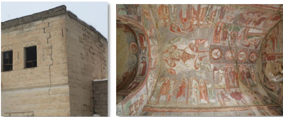
Figure 11. Crack in the facade wall, Figure 12. Crack in the vault of Çavuşin Church (Aktaş, 2019)
