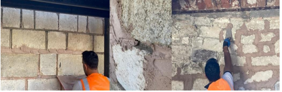
Figure 42. Consolidation of the masonry and joint mortars in the walls, the Restoration of Macedonia Tower, Edirne, 2024, (Osmanoğlu & Köse, 2024)
