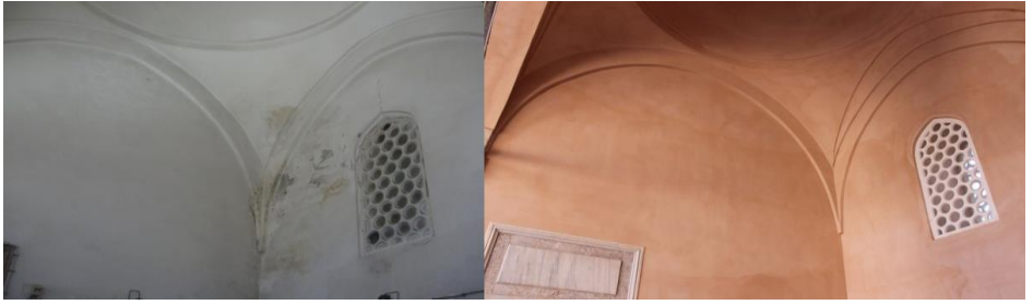
Figure 24. Repair of the iwan walls with the original mortar, rough plaster, and finish plaster as recommended in the material report, Restoration of Tabhane Building of Süleymaniye Complex, Istanbul, 2012-2018, (Osmanoğlu, 2015)
