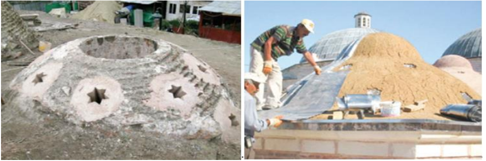
Figure 2. Integration of the eye-shaped openings in the warmth dome and lead covering application, Restoration of Bayezid II Bath, Istanbul, 2005-2014, (Osmanoğlu, 2008)
