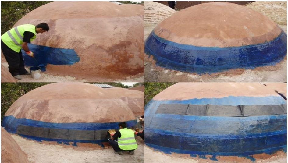
Figure 9. Reinforcement application using carbon fiber tape on the domes, Restoration of Darüşşifa Building of Süleymaniye Complex, Istanbul, 2009-2016, (Osmanoğlu, 2012)
