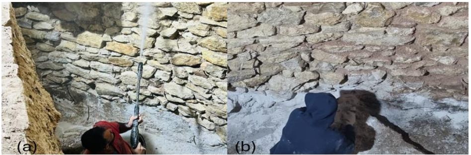
Figure 41. (a) Cleaning of the foundation walls with high-pressure water and (b) application of hydraulic lime injection to the walls, the Restoration of Macedonia Tower, Edirne, 2024, (Osmanoğlu & Köse, 2024)
