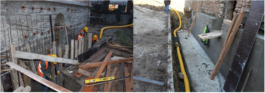
Figure 39. Strengthening the existing foundation by widening it with the construction of an additional reinforced concrete band wall, the Restoration of Akşemsettin Primary School, Istanbul, 2013-2016, (Osmanoğlu, 2013)
