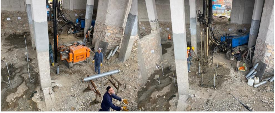
Figure 34. Strengthening the building foundation through micro-pile applications, Restoration of the Building No. 5, Haydarpaşa Train Station, Istanbul, 2017-2024, (Osmanoğlu, 2017)
