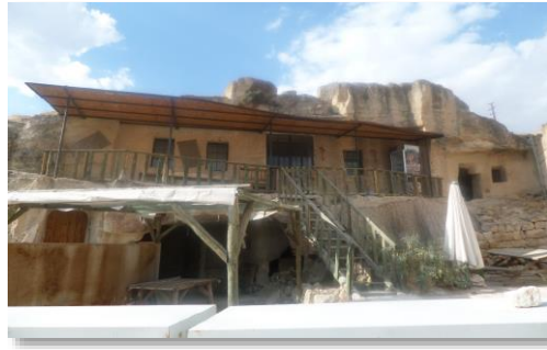
Figure 16. The building added to the Church of St John the Baptist
