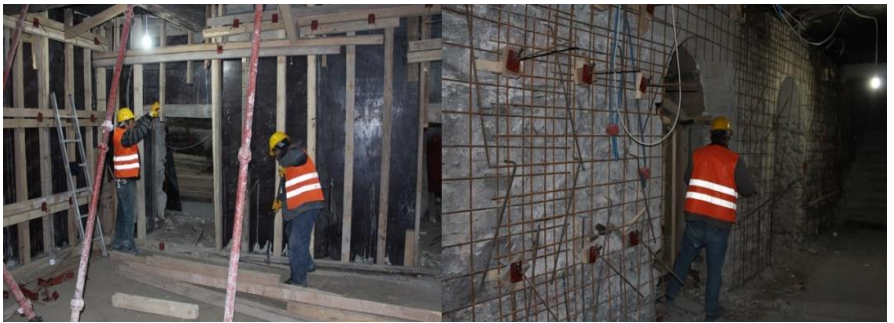
Figure 40. Application of sprayed concrete onto the steel mesh reinforcements anchored to the existing load-bearing walls, the Restoration of Akşemsettin Primary School, Istanbul, 2013-2016, (Osmanoğlu, 2013)
