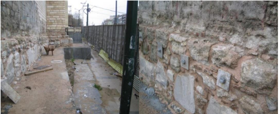
Figure 4. Anchorage application with connection bars on the inner and outer sides of the foundation walls on the south facade, Restoration of the Bayezid II Bath, Istanbul, 2005-2014, (Osmanoğlu, 2007)
