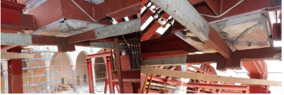
Figure 18. Cleaning and painting the ties with anti-rust paint, Restoration of Tabhane Building of Süleymaniye Complex, Istanbul, 2012-2018, (Osmanoğlu, 2014)
