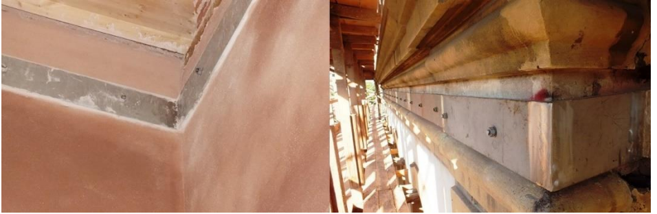
Figure 29. Application of stainless steel ties to strengthen the walls of the building, Restoration of Fatih Sultan Mehmet High School, Istanbul, 2010-2017, (Osmanoğlu, 2016)
