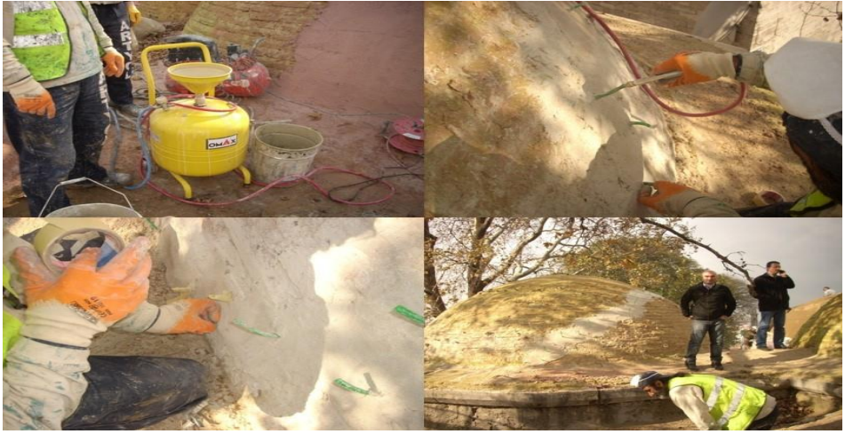
Figure 8. Stages of hydraulic lime injection application for dome cracks, Restoration of Darüşşifa Building of Süleymaniye Complex, Istanbul, 2009-2016, (Osmanoğlu, 2012)
