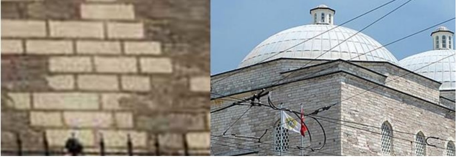
Figure 5. Stitching of the deterioration in the external facade wall masonry and consolidation application with binding mortar on the walls, Restoration of the Bayezid II Bath, Istanbul, 2005-2014, (Osmanoğlu, 2007)
