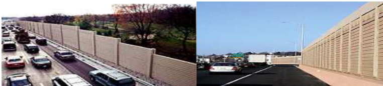
Figure 13. Use of sound absorbing materials made of concrete and metal on highways
