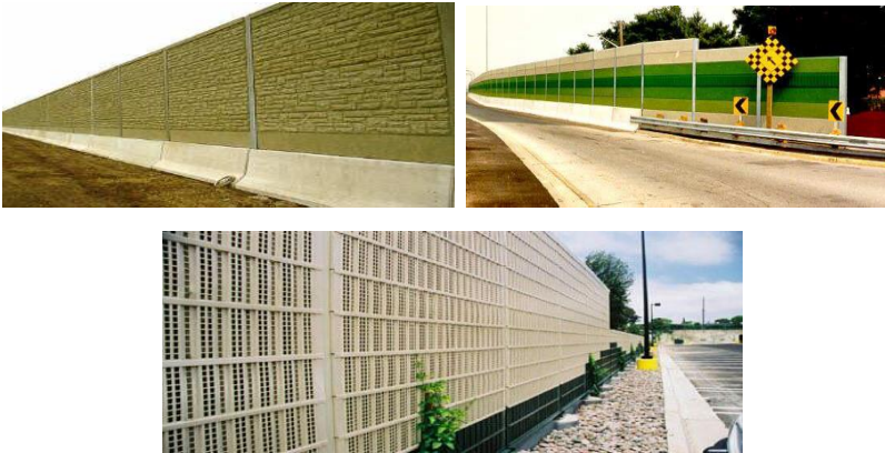
Figure 9. Examples of artificial sound absorbing materials
