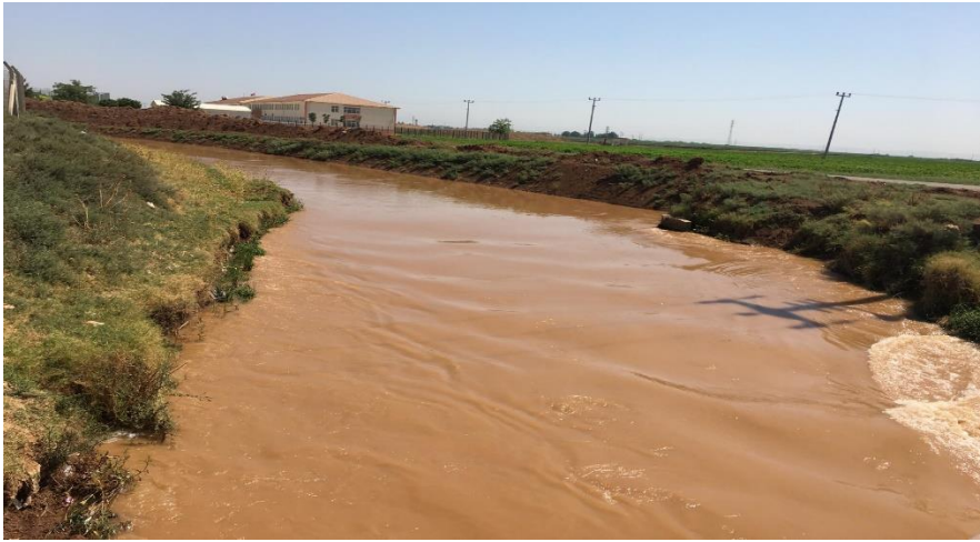
Figure 3.2. Harran Plain Arican Main Drainage Canal
