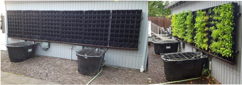
Figure 2: Hydroponic panel system application - California / USA (Url-1).
