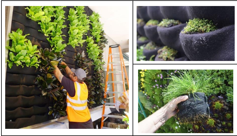
Figure 3: Felt system application- San Francisco / USA (Url-2).
