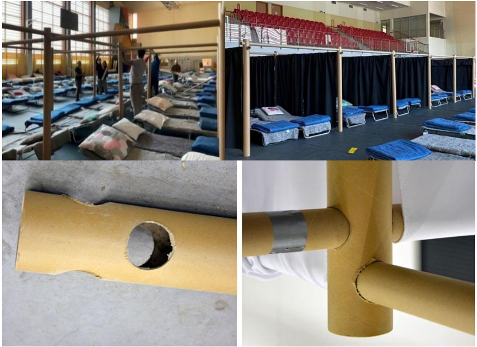
Figure 10. Refugee Shelter Modules Designed by Shigeru Ban (Ukraine Refugee Assistance / Paper Partition System, 2022).
