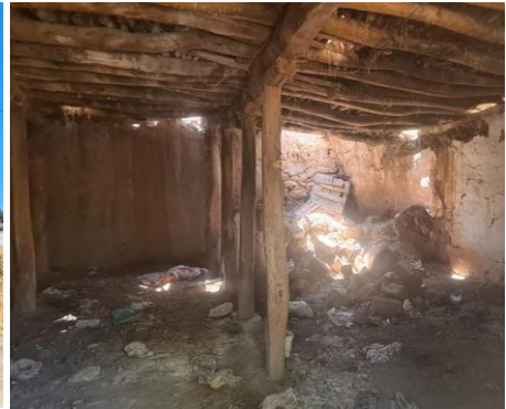
Figure 19. Collapsed Adobe Structures
