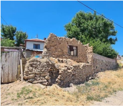
Figure 19. Collapsed Adobe Structures
