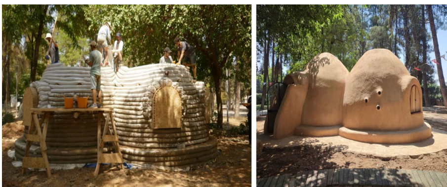
Figure 6. A Superadobe structure, applied in Türkiye in 2024, is shown in both the construction phase and the completed state (Cansız, 2024)
