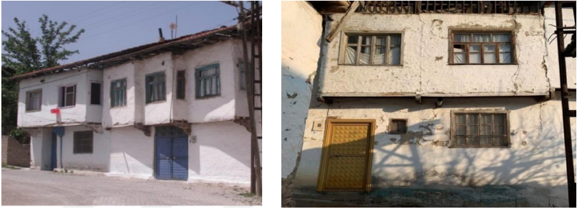
Figure 3. Examples of mud-brick-filled structures in Malatya (Can, 2020)
