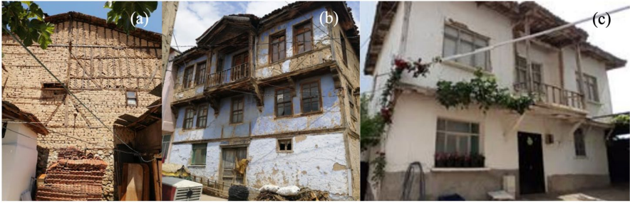
Figure 4. a, b and c) examples of traditional Turkish houses in the village; mud-brick-filled structures (Doğan Talyak, 2021)
