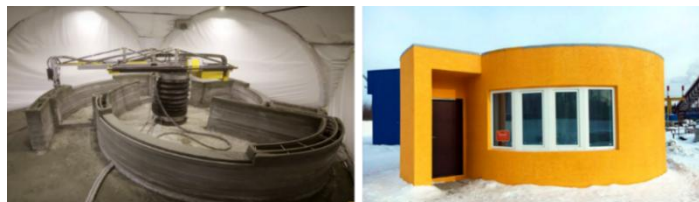
Figure 9. Residential Unit Produced by Apis-Cor (Sakin & Kiroglu, 2017).
