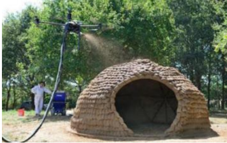
Figure 11. Bio-Spraying of Mortar onto Building Envelope (Šamec, et al., 2019).
