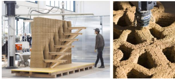
Figure 8. Wall Created with 3D Printing (Gomaa et al., 2022).
