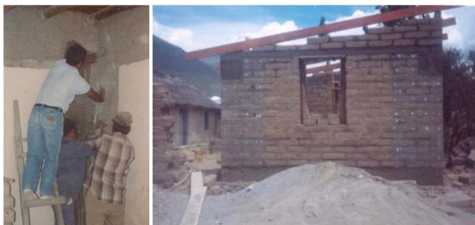
Figure 1. Installing Vertical Mesh Strips at Corners (Quiun, 2009).
