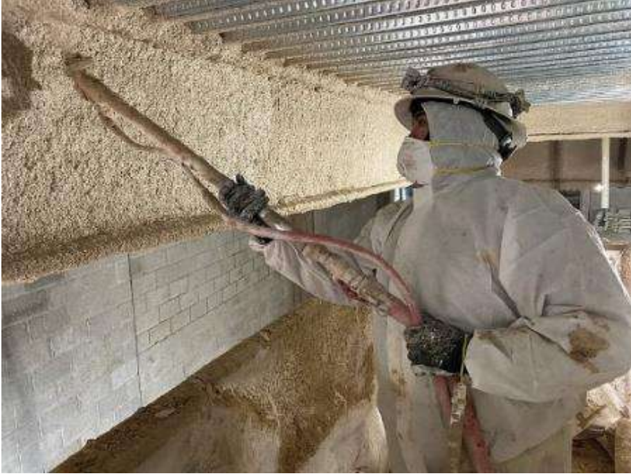
Figure 1. Spray coating application
