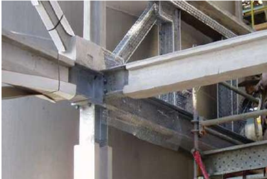
Figure 2. Fireproof-painting for fire stopping.
