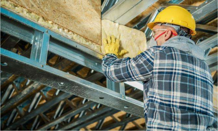
Figure 9. Stone wool (rockwool) application on steel.
